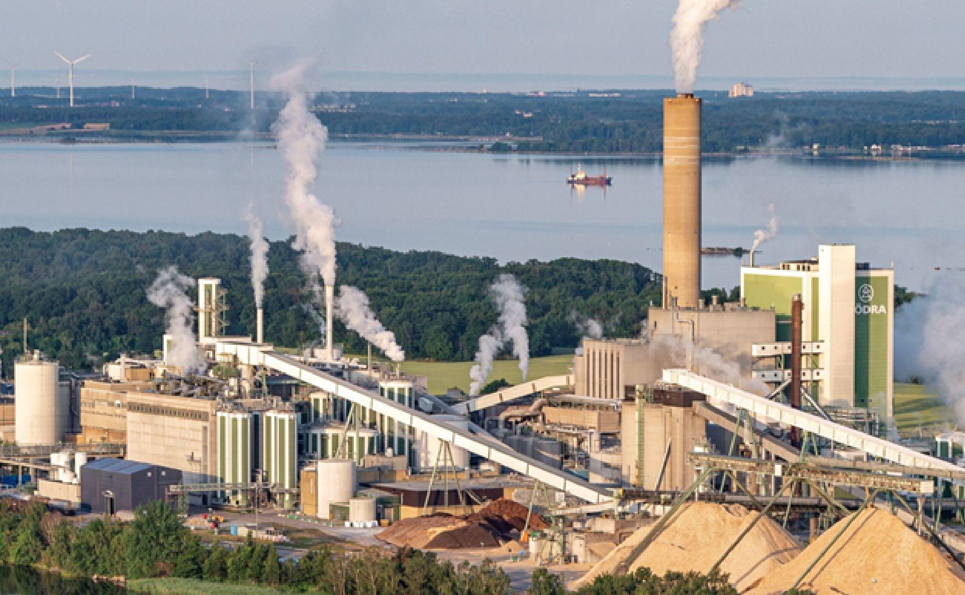
Figure 3: Södra's mill in Mörrum, Sweden. Courtesy: Lenzing Group
