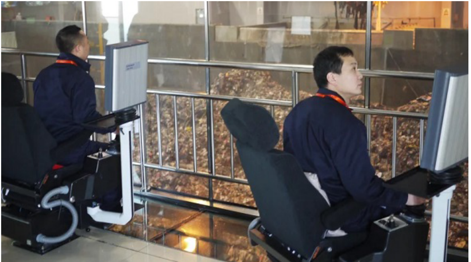
Figure: Engineers at Beijing's Gao'antun incinerator power plant control giant claws with joysticks on special chairs inside a cockpit. The claws are capable of lifting eight tons of garbage with each scoop. Courtesy: Rob Schmitz/NPR
